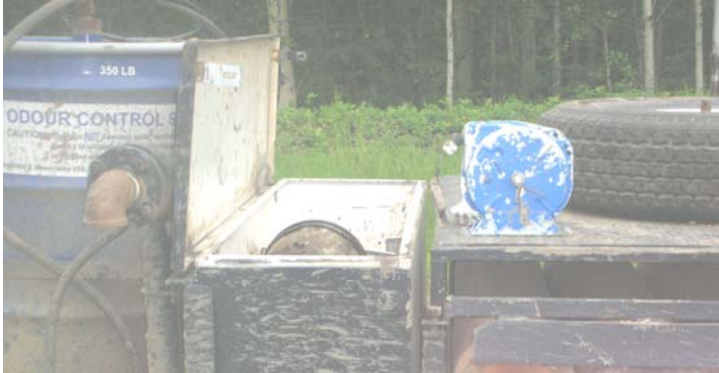
Lid was not secured in the open position ↑
