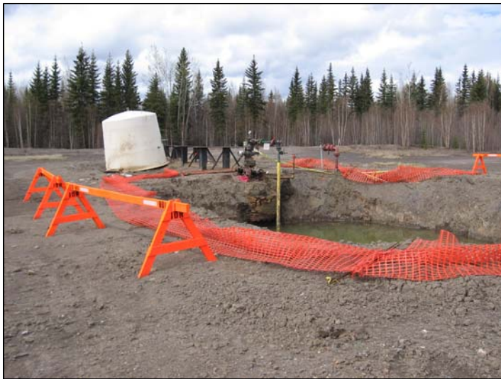
Condition of site at time of inspection
